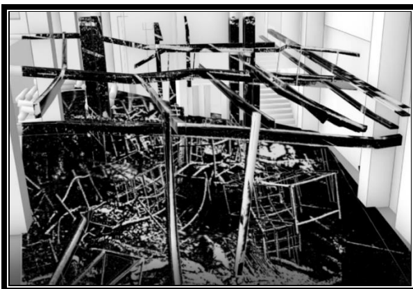
Fig 6. Timber structure with twisted steel beam
